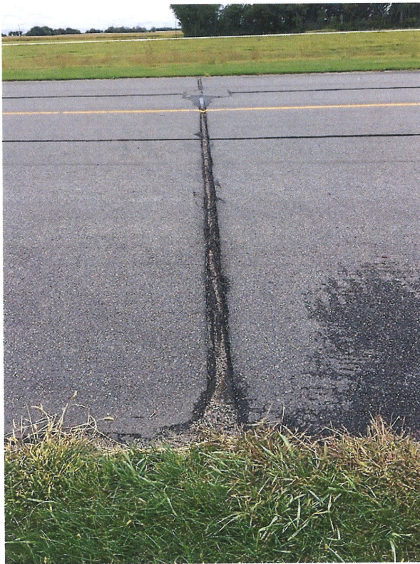
Taxiway Pavement Joints, 5-inches Wide
