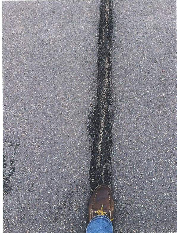
Taxiway Pavement Joints, 5-inches Wide
